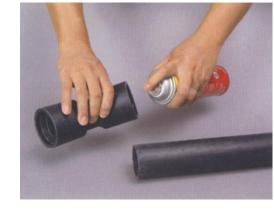
Spray the rubber inside the joint with wax or soapy water (to increase its lubricity)
