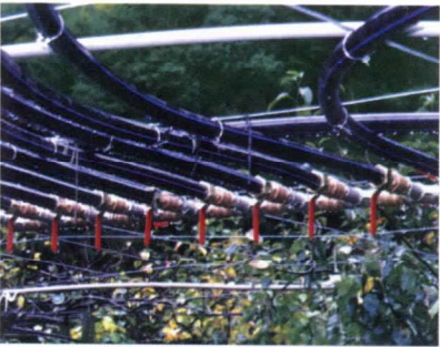
山區灌溉系統工程 Irrigation system engineering work in mountain areas.
