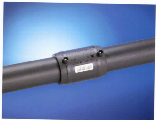
電焊套另件施工完成圖 Completion of Electrofusion Fitting.
